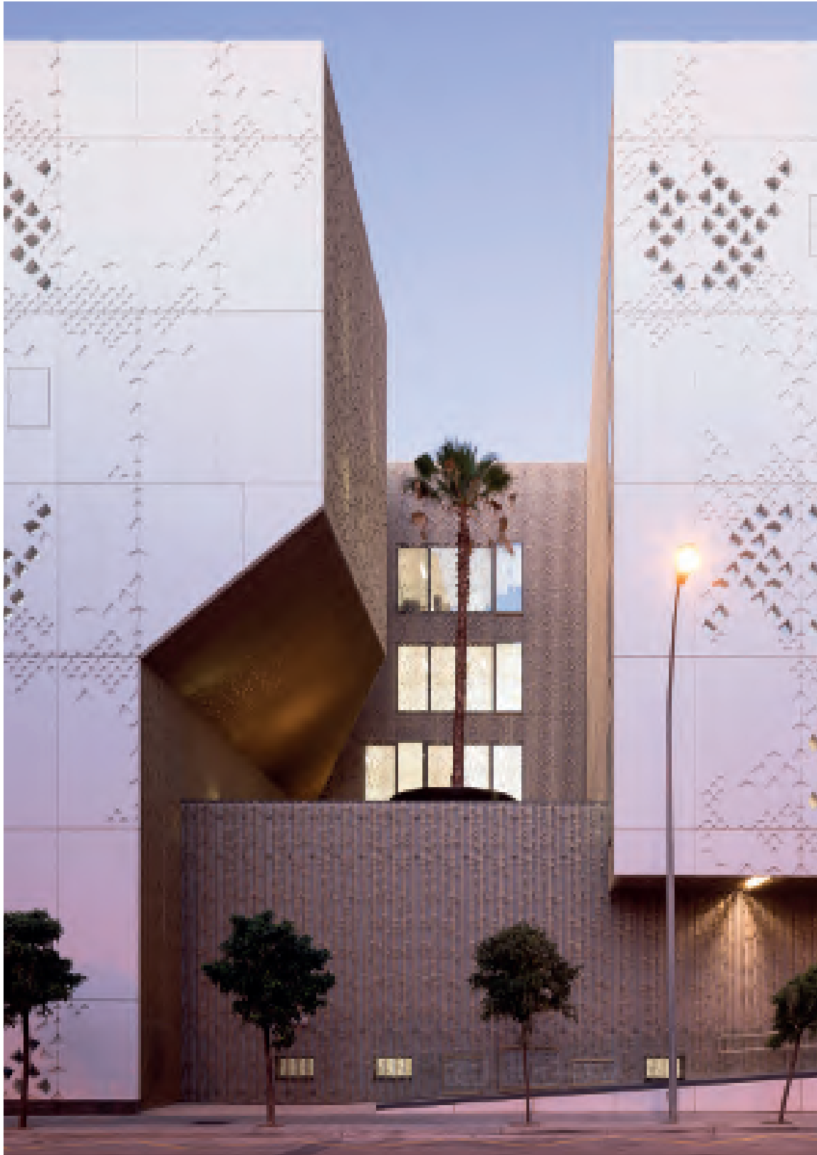
Palace of Justice, Córdoba, Spain Architects: Mecanoo and Ayesa Photographer: Fernando Alda
